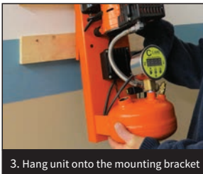
3. Hang unit onto the mounting bracket
