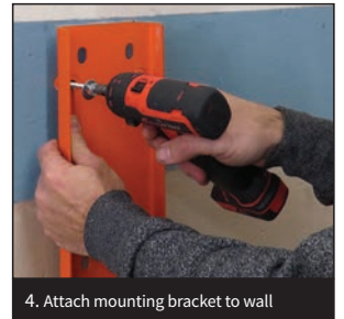
4. Attach mounting bracket to wall
