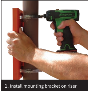
1. Install mounting bracket on riser
